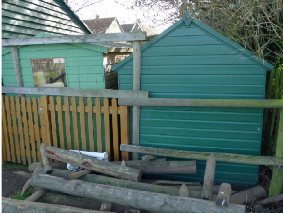
Shed 02 & 03 (Rear Elevation)
